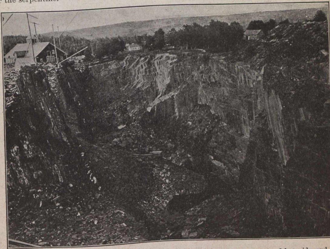
Fig. 1.—New Rockland Slate Quarry, Looking Northeast. This quarry is some 799 feet in length, 75 feet wide, and nearly 200 feet deep. The cleavage the of slate dips at a high angle to the Southeast.
