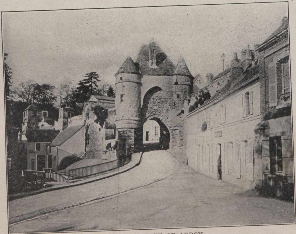
LAON.—THE GATE OF ARDON.
