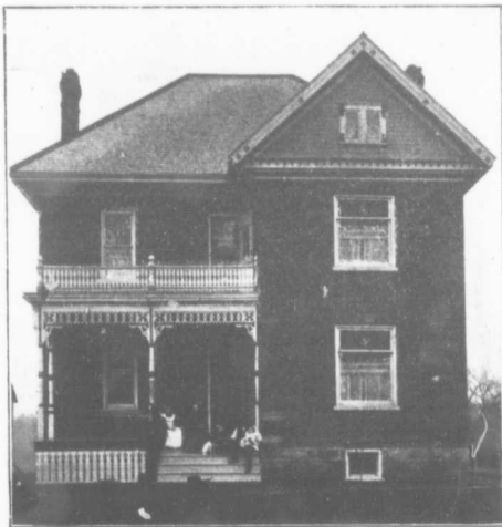
RESIDENCE OF MR. JOSEPH McDONALD, HURON CO., ONT.
