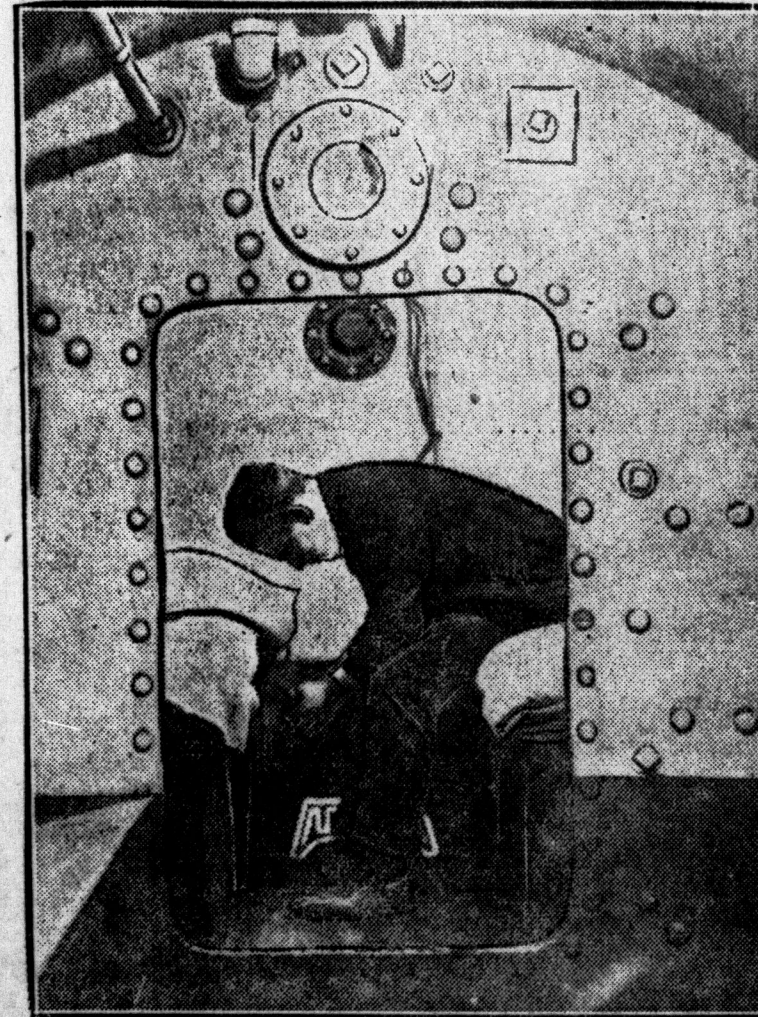
Sixty-five per cent. of the Hudson River vehicle tunnel has been completed. The pressure chamber is shown in which workmen are tested and also treated when seized with cramps due to emerging too quickly from the high pressure
