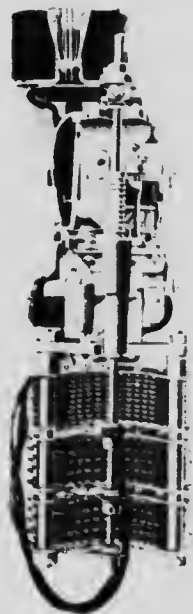
AN ENLARGED VIEW OF A SUBSCRIBER'S AUTOMATIC TELEPHONE CONNECTOR.
