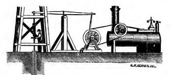
Machinery used in Boring Petroleum Wells.
