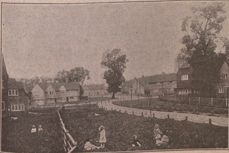
GOVERNMENT HOUSING SCHEME AT WELL HALL, WOOLWICH
