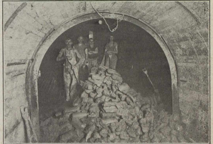
Fig. 9.—Showing Method of Excavating and Nature of Material, Section 2.
