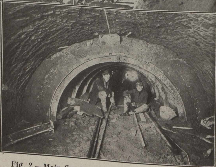
Fig. 2.—Main Garrison Creek Storm Overflow Sewer, Showing the Use of Steel Forms for the Invert.
