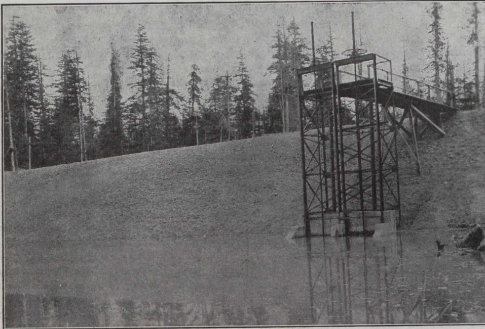
The Intake Tower in Forebay Reservoir.
