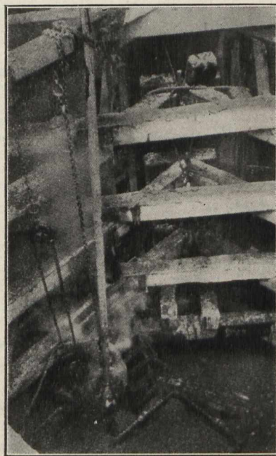
Interior of Shell on Pivot Pier, Showing Bracing.
