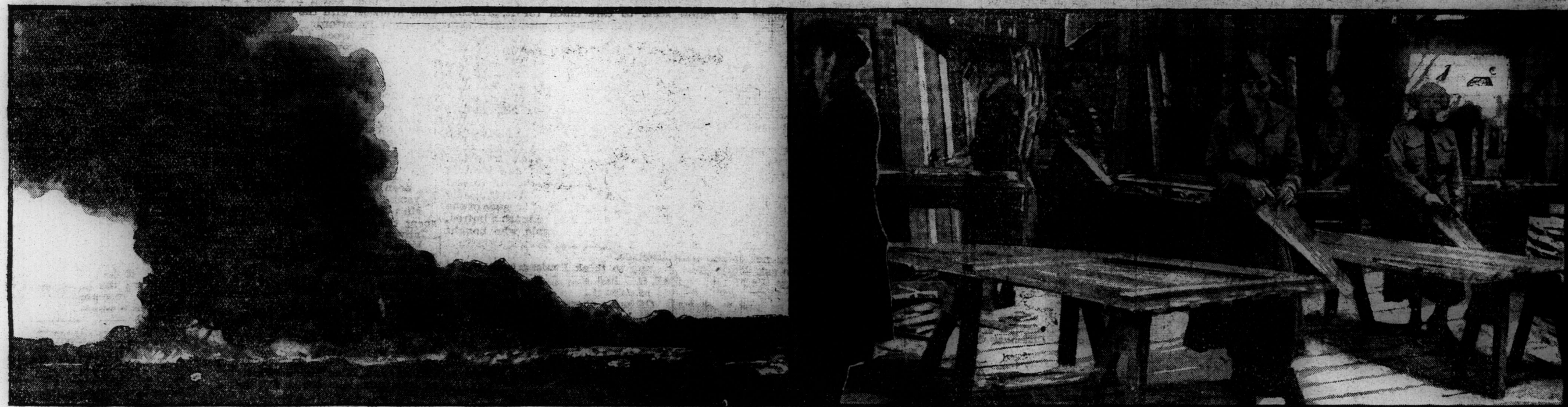
On the British Western Front.—What the Queen saw.
