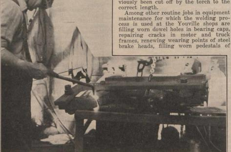
Fig. 4. Welding New Gear Case Lug on Motor.
