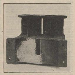
Fig. 3. Repairs to Air Compressor Crank Case.
