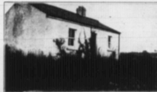
An Irish laborer's cottage built with the assistance of the government.
