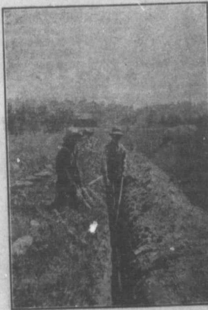
Mr. Dawson Grading a Ditch Bottom.
