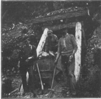
ENTRANCE TO A YMIR MINE, BRITISH COLUMBIA.
