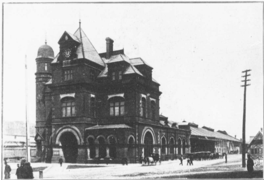
Intercolonial Railway Station
