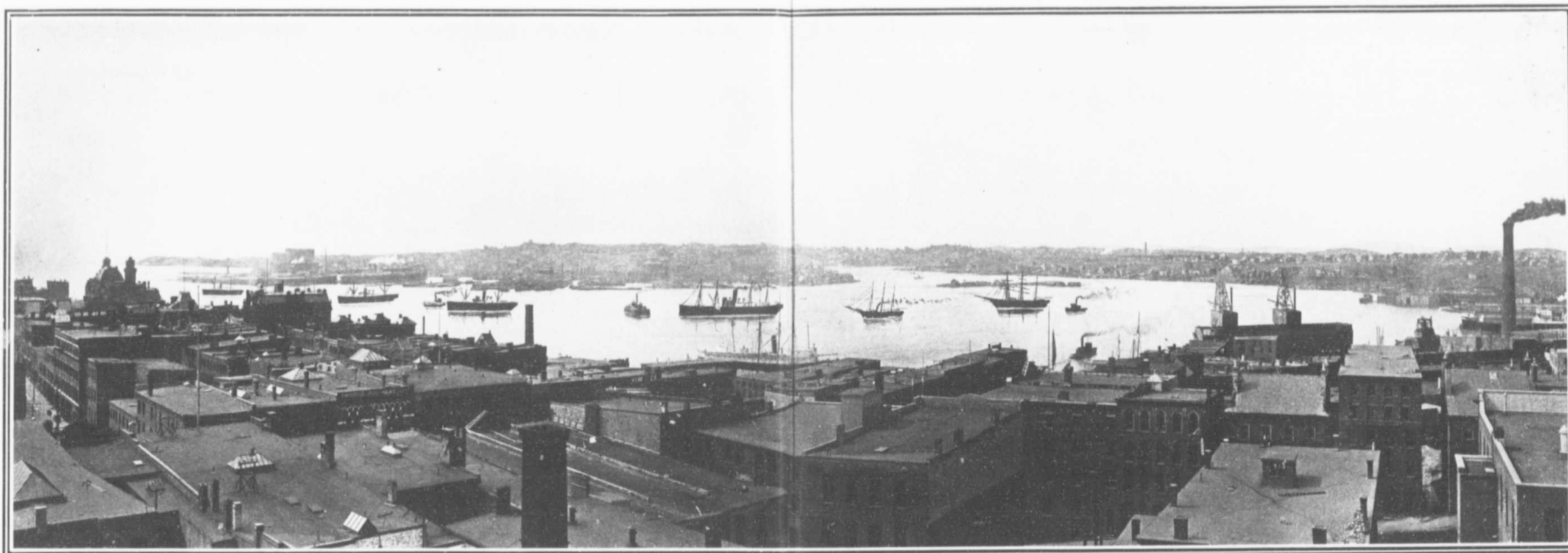
View of St. John Harbor from Emerson & Fisher Building.
