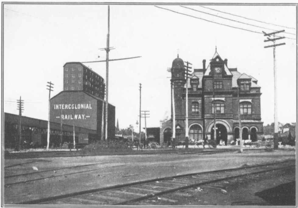
Intercolonial Railway Depot and Elevator.
