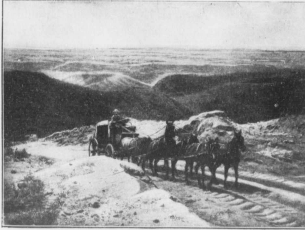
Transportation by stage-coach. In many hilly and mountainous regions the stage-coach has to be used. Notice the ridges which aid the horses in getting a firm footing.
