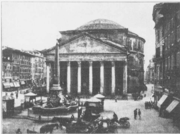
A square in Rome, showing the Pantheon, built in 27 B.C. The finest and best preserved work of Roman architecture.
