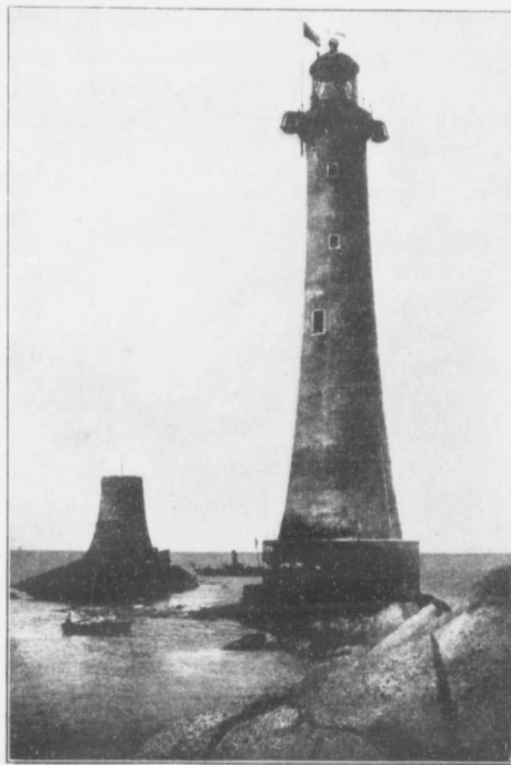
Eddystone Lighthouse marks a dangerous rock off the south-west coast of England.
