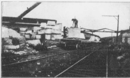
Unloading stone brought from a quarry, where it was cut into blocks, placed on flat cars, and shipped to its destination.
