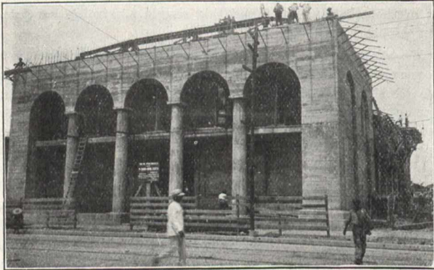
Front View, Bank of Nova Scotia, August, 1907.
