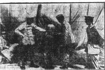
HUNS OVERHAULING A GERMAN "SAUSAGE" Observation balloons, called "sausages," are delicate things to handle, but owing to hard service must often be inspected. Inspection is made of the inside and outside of the envelope. Our photo shows officers and soldiers in the "sausage" inspecting the inside.
