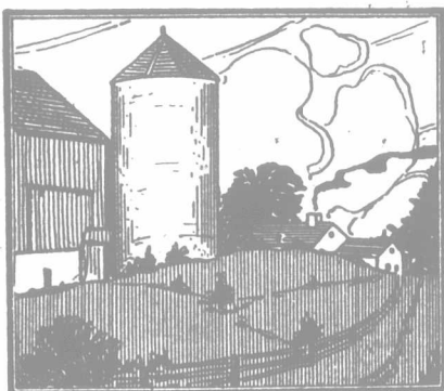
C ONCRETE is the ideal material for barns and silos. Being fire, wind and weather proof, it protects the contents perfectly.
