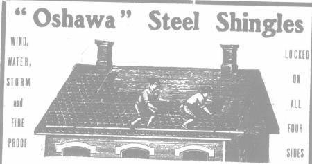
Made from Painted or Galvanized Steel at prices varying from \$2.85 to \$5.10 per 100 square feet, covering measure. This is the most durable covering on the market, and is square feet, covering measure. This is the most durable covering on the market, and is an ideal covering for Houses, Barns, Stores, Elevators, Churches, etc. Any handy man can lay the "Oshawa" Shingles. A hammer and snips are the only tools required.
