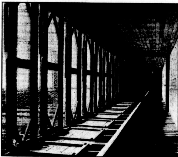
Inside View of Winter Brooder House, Glenavy Farm.
