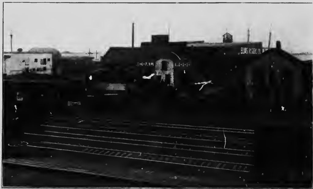
ONE OF THE SIX YARDS OF THE ELIAS ROGERS CO. Toronto, Canada
