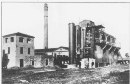
Mond, by-product recovery peat producer-gas power plant at Orentano, Italy.
