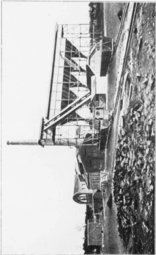
3,000 horse-power, by-product recovery peat producer-gas power plant on the Schweizer Moor; view showing fuel bins, hoppers, and loading device.
