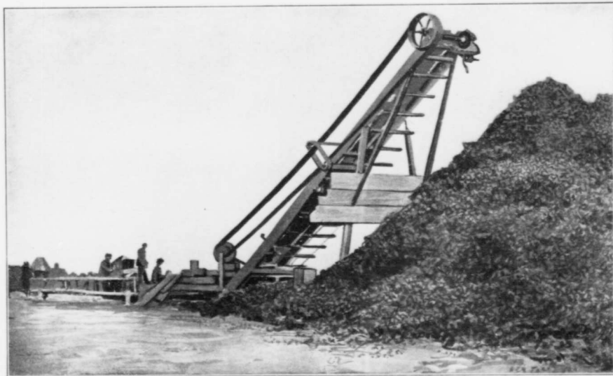
Peat elevator in operation.
