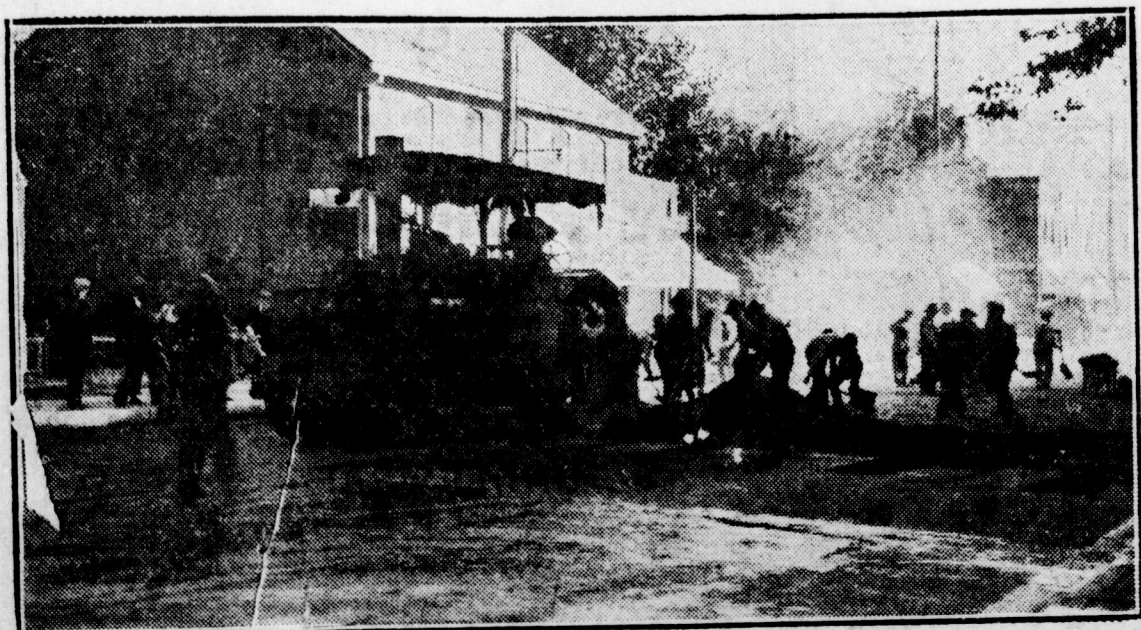
The recent paving of Elizabeth street, Barrie, Ontario, is a big improvement to the main highway from Toronto north, to Barrie, Orillia and Muskoka. The citizens held a street dance to celebrate the completion of the work
