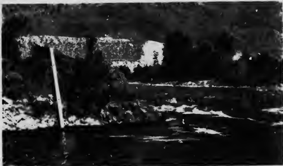
Nicola river, at mouth. Inclined staff gauge bolted to solid rock.
