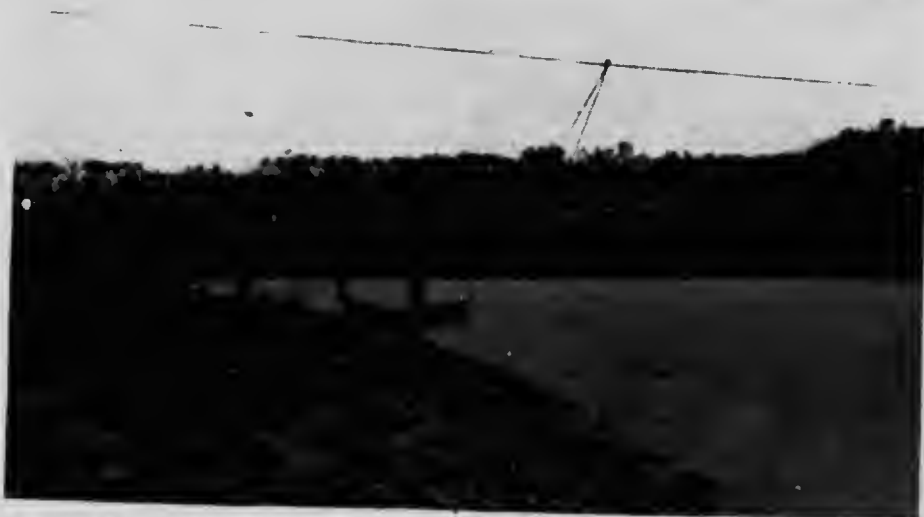
Chain gauge and measuring section, on Skeena, at Hazelton. Measurements are made from the Indian dugout canoe shown in the foreground, points of observation being marked by a tag line.
