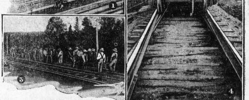
1 Unloading new rail from a flat car. 2 A Canadian Pacific work train. 3 Placing a new rail unit. • 4 Throwing the old rail to the outside of the track. Note how the wheels are edging the old metal over the new.
