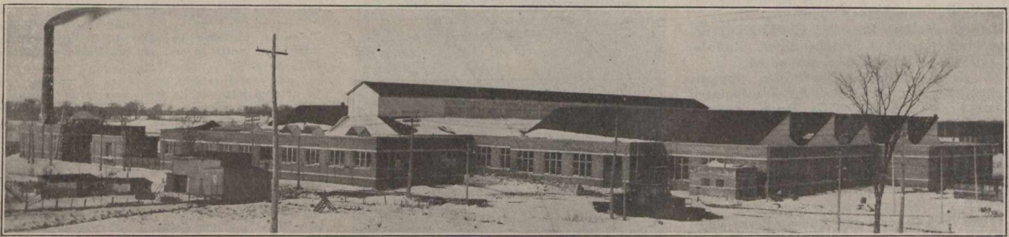
Fig. 1.—Montreal Tramways Co.'s New Plant, viewed from the South.
