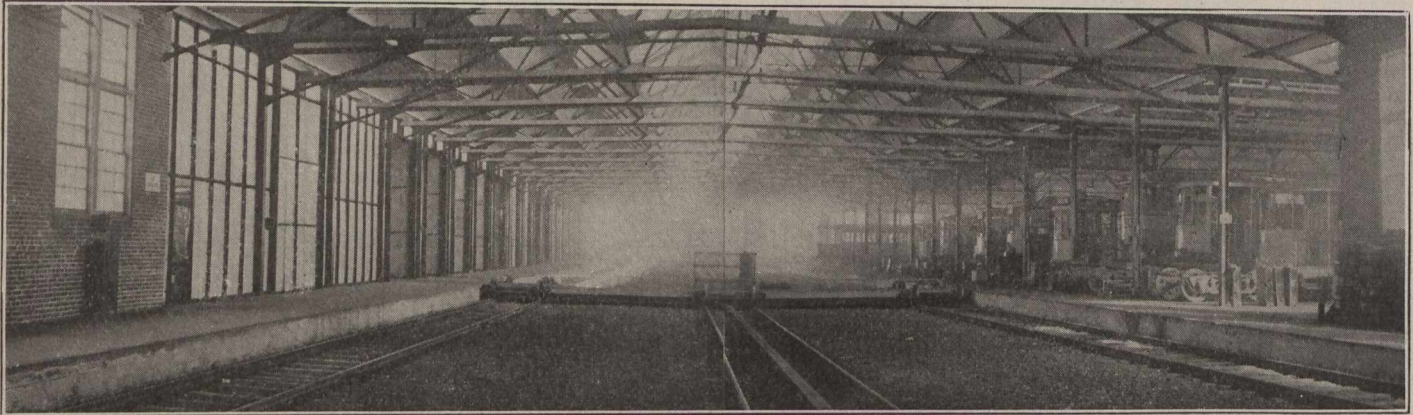
Fig. 4.—Covered in Transfer Table which centrally divides the Shops.
