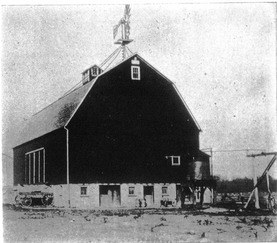
Stock barn of Mr. John D. Ferguson, in the township of Yarmouth. Dimensions of the building, 80 x 48 feet; foundations of concrete, 2 1/2 feet deep. Floors and root cellar all of Thorold Cement.
