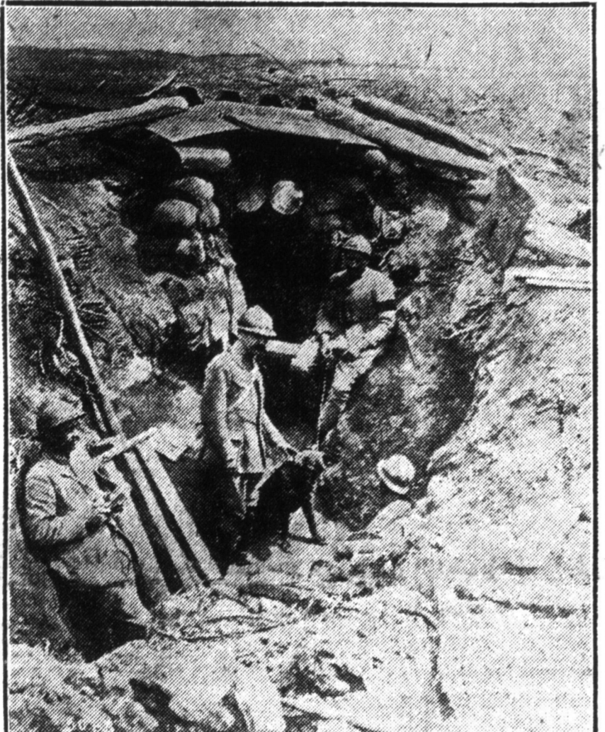
A French observation post, in advance of the front line trenches on the Aisne, and its occupants. Note the heliograph in the shelter. This is used to signal results of artillery fire to the trenches, some distance back. The dog is a courier.
