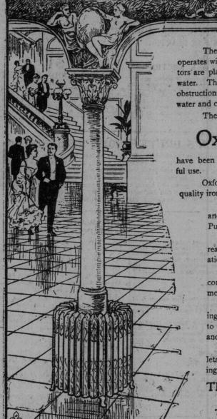
The Oxford Hot Water System of heating operates with perfect silence as the Oxford Radiators are planned to give a clear passage for the water. They do not contain diaphragms or other obstructions in the water passages to check the water and cause the system to be noisy. The efficiency and durability of
