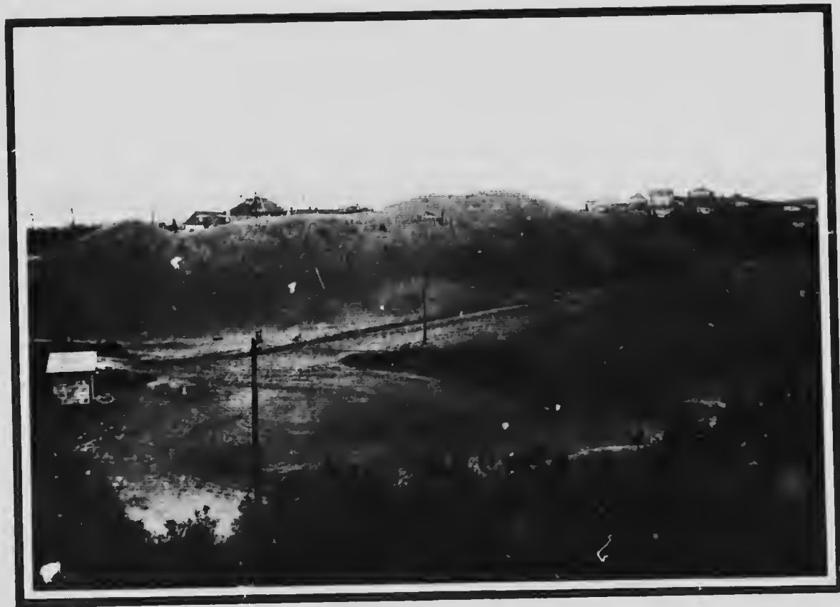
BUFFALO MINES, LIMITED—Big dump of mill tailings on the property. The mountain of sand from the low-grade mill shown above contains between 300,000 and 400,000 tons, and it will be treated by the new oil flotation process, recently installed, with a capacity of 500 tons daily. The tailings are estimated to contain from 4 to 7 ounces of silver per ton.
