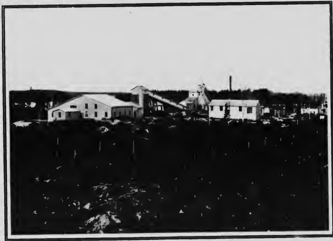
TECK-HUGHES MINING COMPANY, LIMITED, KIRKLAND LAKE. General view of the mill and plant. The mill has a capacity of 500 tons daily and the cyanidation system is used, counter current decantation. During the present summer a new 12-drill compressor was installed. Controlling interest in the Company is owned by Mr. C. L. Demson and associates of the Buffalo Mines, Cobalt, and the property is under the same management.
