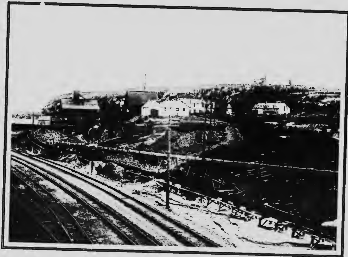
LaRose Consolidated Mines, Limited. Main property of the Company, where Fred LaRose, the railway blacksmith, found silver during the construction of the T & N. O. railway. The LaRose Company also controls the Lawson, University, Princess, Fisher-Epelt and Violet properties. Total production of the LaRose properties to the end of 1915 has been 22,891,037 ounces, valued at $11,514,043.70. Dividends paid to January 20, 1916, including profits to original owners, $6,907,409.56.
