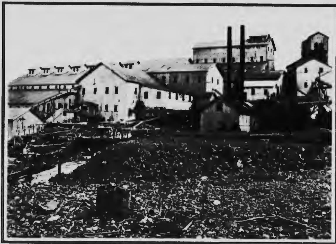
NIPISSING LOW-GRADE MILL.—The big low-grade mill of the Nipissing Mining Company, Limited, erected at a cost of $375,000. This plant is equipped with 40 stamps, and has a daily milling capacity of 300 tons. During the year 1915 the mill treated 77,183 dry tons, and the bullion recovered from this tonnage totalled 2,127,372 ounces, an extraction of 87.52 per cent. The cost per ton, including transportation of ore and picking plant, was $3.913. The system of concentration used is cyanide. Ore from the 4th of July shaft, a mile away, is transported by aerial tramway to the mill.
