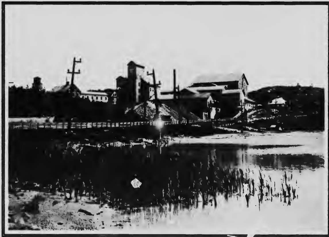
THE DOMINION REDUCTION COMPANY, LIMITED: Operating the mining property formerly known as the Nova Scotia. The mill on the property is equipped with 40 stamps and has a rated capacity of 200 tons per day. The Company treats ore in its mill for the Crown Reserve Mine, the Comet, Drummond Fraction and the Kerr Lake Mines. During 1915 the mill treated approximately 78,300 tons, from which 1,500,000 ounces of silver were recovered.
