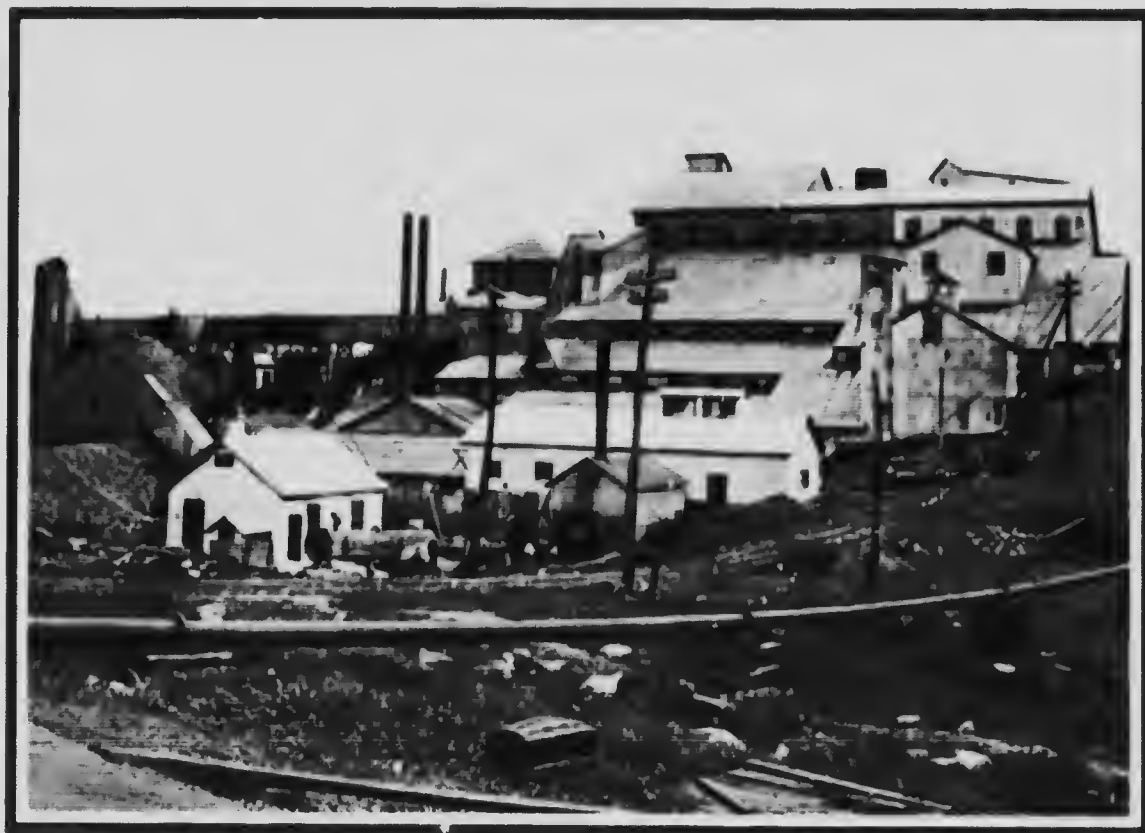
General view of the McKinnon Damaged Silver Mining Company's Mill and Mine Buildings. The mill has a capacity of 400 tons a day and in the spring of 1916 the first of flotation plant to be installed in Northern Ontario was put in operation. The latter plant is used to treat the tailings and thus obtain a higher recovery. The Company to the end of 1915 had paid 20 1/2% in dividends on the capital stock of $2,500,000, or a total of $5,000,751.
