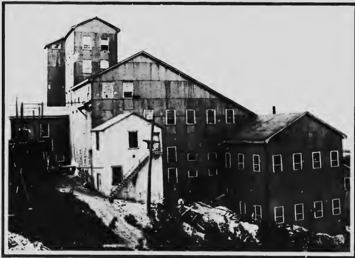
Mill of the O'Brien Mine. Equipped with 20 stamps, having a capacity of 200 tons per day. During 1915 the mill treated 52,883 tons, recovering therefrom 526,272 ounces of silver. The process at the O'Brien mine is cyanide treatment, the plant being the first cyanide mill in Cobalt. The sodium sulphide method of precipitation was originated here.
