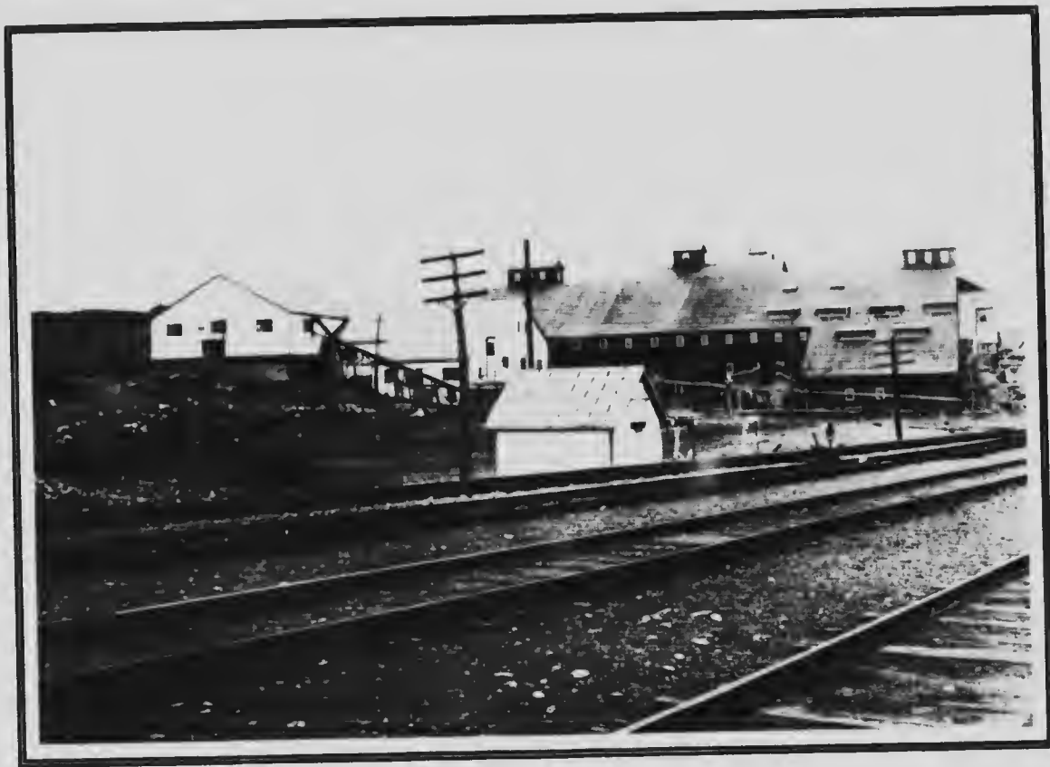
MILL OF THE COBALT REDUCTION CO. MINING CORPORATION OF CANADA, LIMITED, showing new cyanide addition to the left. This mill was built in 1907, under the name of the Muggley Concentrator. Later it was taken over by the Northern Ontario Concentrators, Limited, and by them sold to the Mining Corporation of Canada, Limited, who have made extensions and improvements to the plant. The mill treats ore from the City of Cobalt mine, the Townsite Extension, and the Cobalt Lake mines, all of which properties are being operated by the Mining Corporation. The mill has a capacity of 300 tons daily, of which 175 tons are treated in the low-grade cyanide plant and not concentrated.
