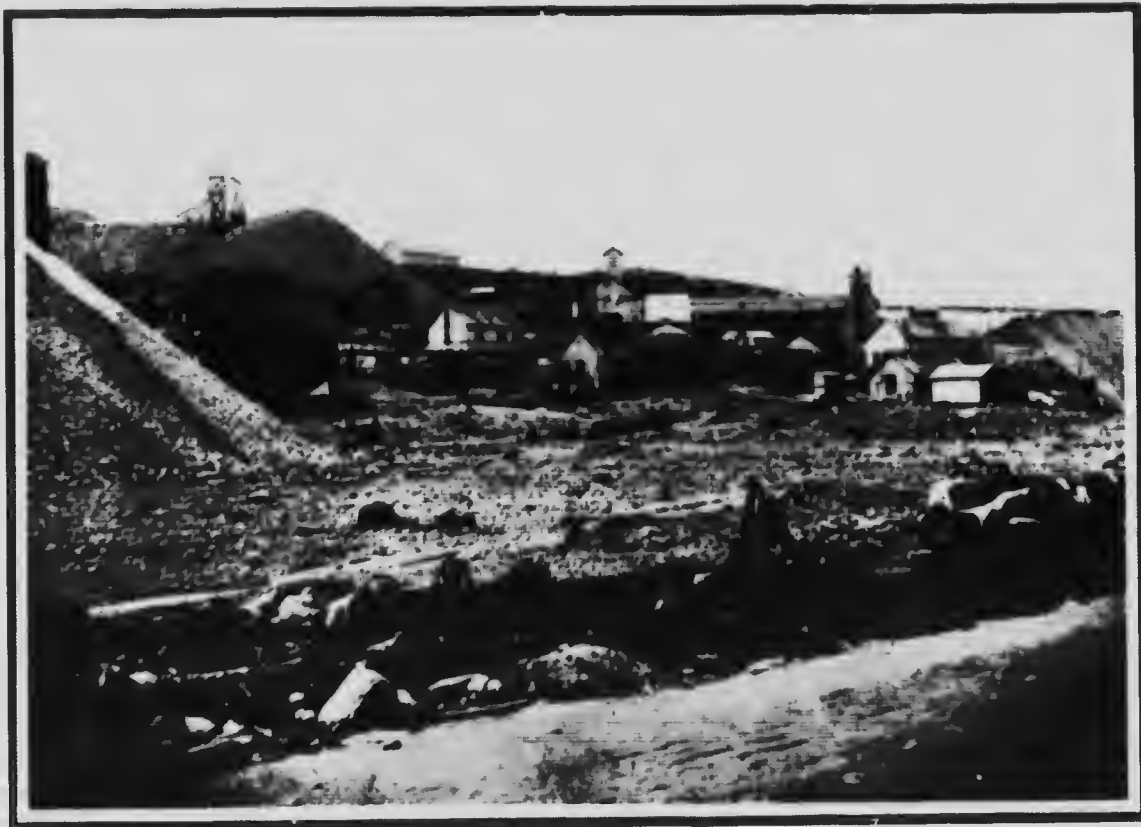
NIPISING MINING COMPANY, LIMITED. Shaft No. 73, one of the best producers of the mine, and the terminal of the aerial tramway.
