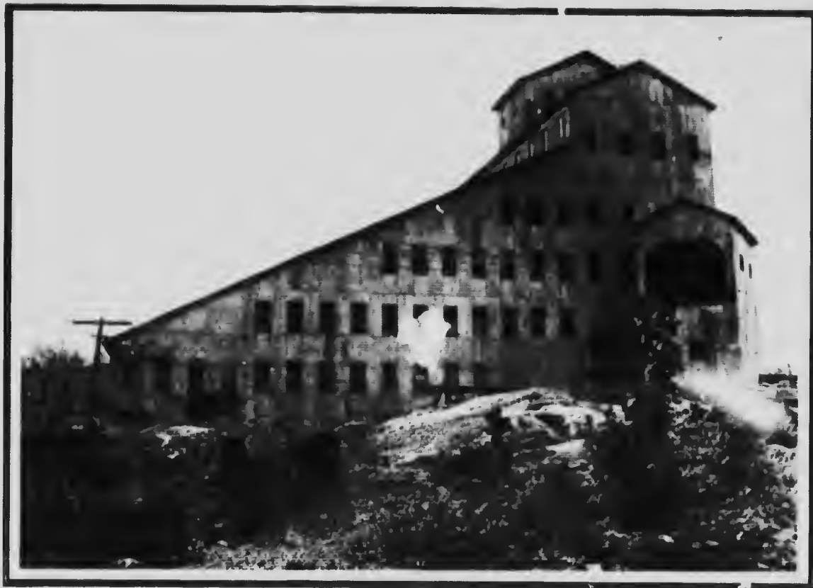
FIG. TEMISKAMING MILL. A 30-stamp, water concentrating mill with a daily capacity of 100 tons of ore. During the year 1913 the mill treated 40,947 tons.
