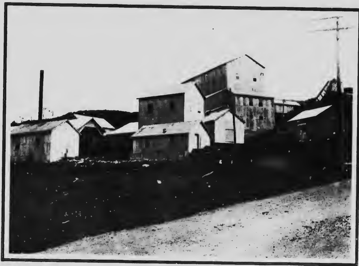
THE FINE NEW MILL OF THE NORTHERN CUSTOMS CONCENTRATORS, LIMITED.—This plant contains 80 stamps, and has a rated capacity of 200 tons per day. The mill treats concentrates, and carries the process further than concentration, returning the concentrates to the mines or shipping them to the smelter on the latter's account. The Company at present handles ore from the Chambers-Ferland, LaRose and Right of Way mines. The mill originally owned by this Company was sold to the Mining Corporation of Canada, and the new plant shown above constructed in 1913-14. An oil flotation plant is to be installed.
