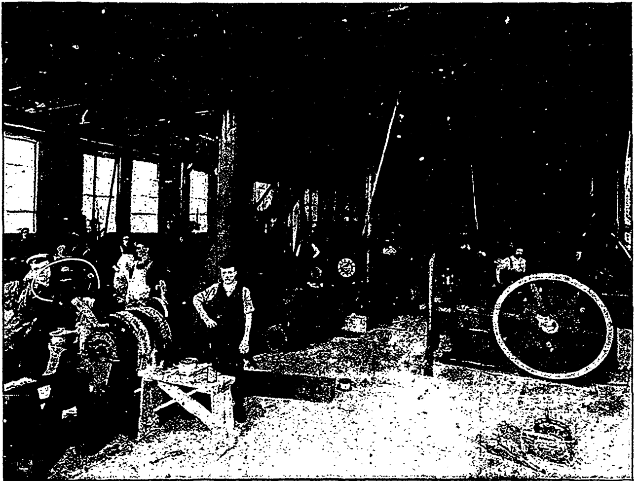
TORONTO ELECTRIC MOTOR CO.'S MACHINE SHOP.
