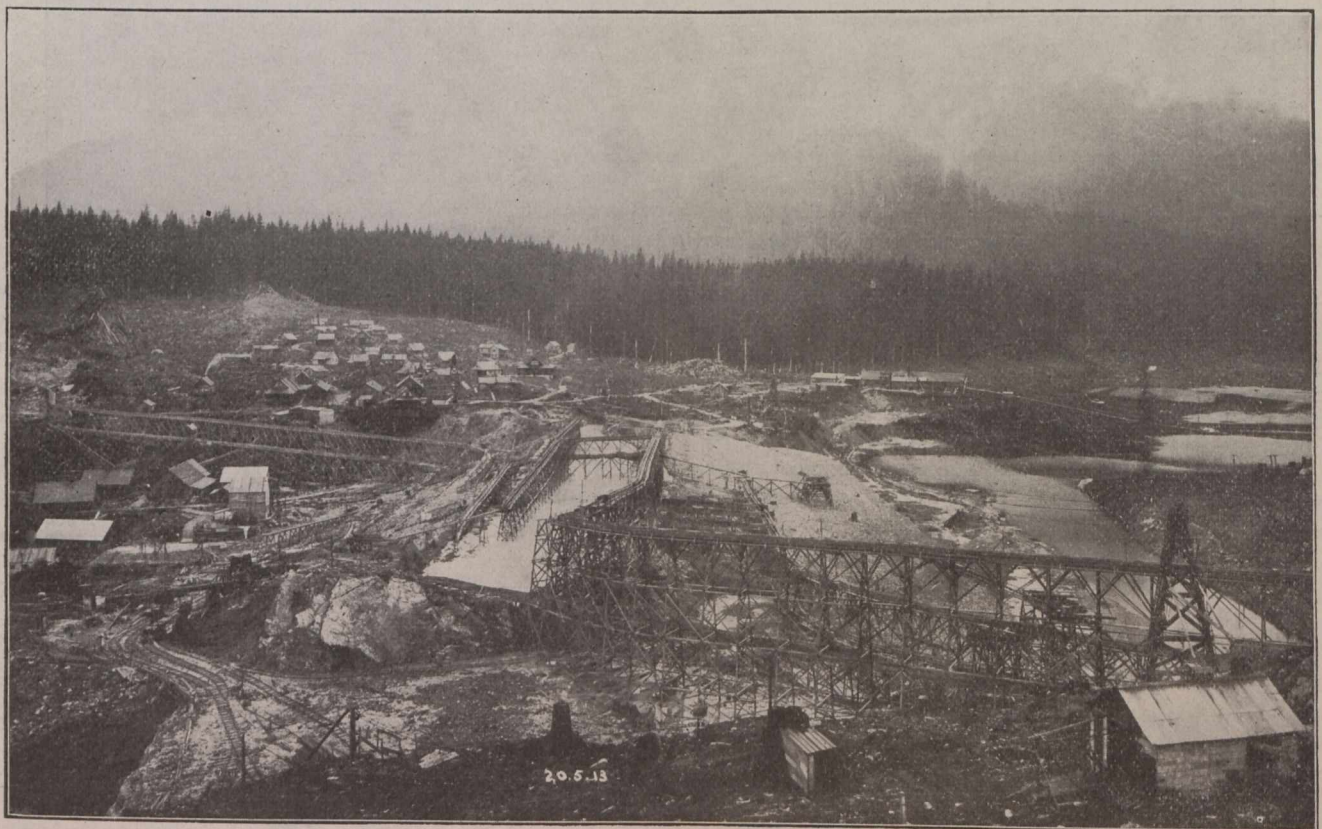
Fig. 1.—General View of Coquitlam Dam During Construction.
