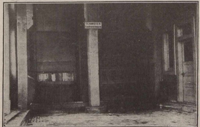
Electric Elevator for Receiving Garbage.
