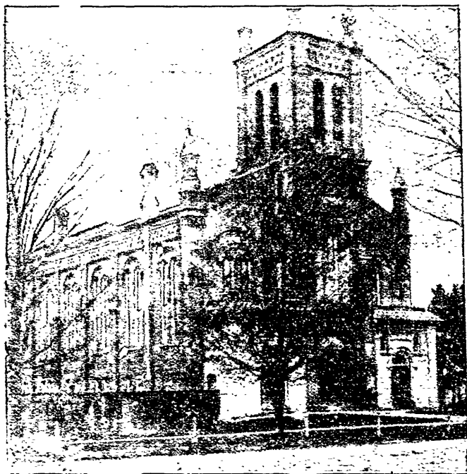
EXTERIOR VIEW OF CHURCH
