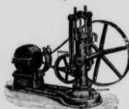
This cut shows a reliable workinghead or pump for shallow or deep wells for e-lectric or Gasoline engine power.
