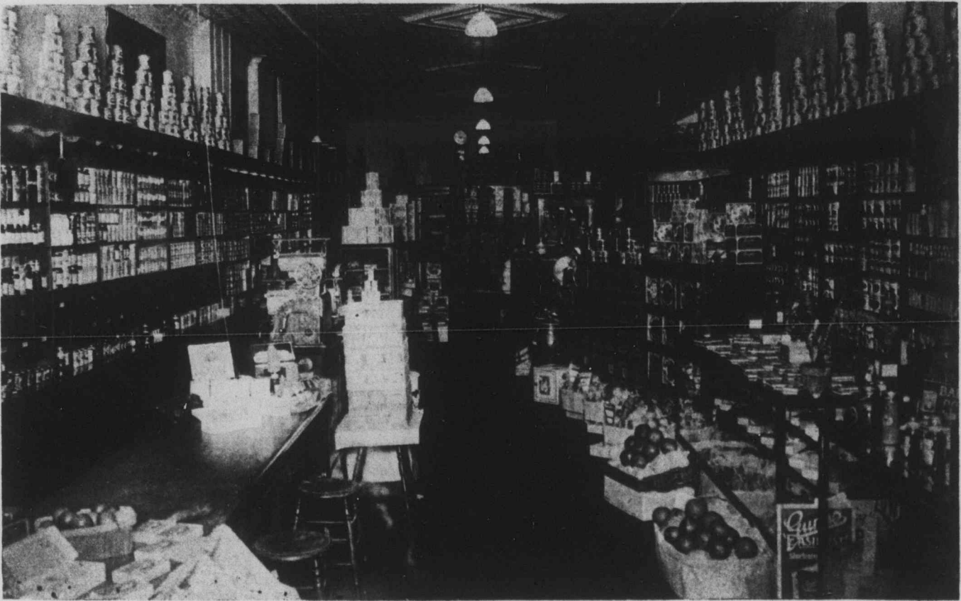
Interior of the R. E. Powell Store, Elgin Street, Ottawa.
