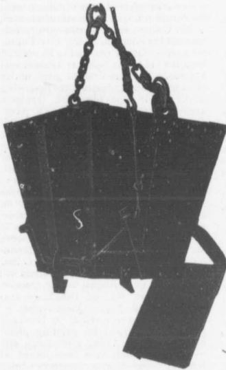
Cyclopean Concrete Buckets.
