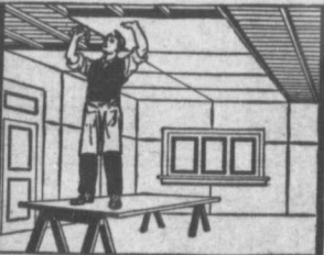
Applying Bishopric Lath Board to Ceiling.
