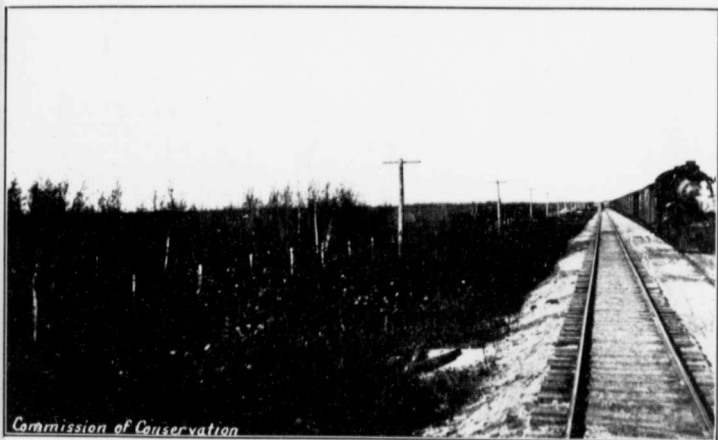
RIGHT OF WAY IN SOUTHEASTERN MANITOBA BADLY IN NEED OF CLEARING
