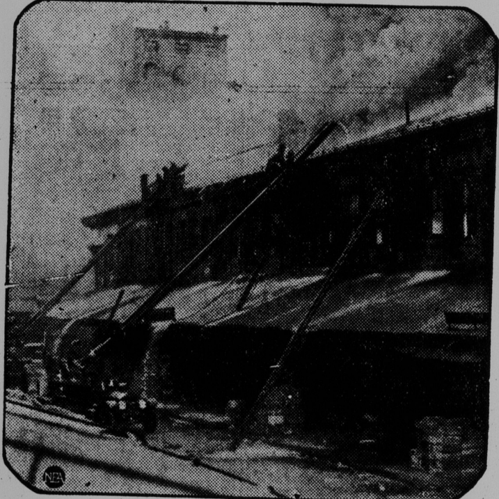
The historic Quincy Market in Boston, Mass., was swept by flames. Practically all apparatus in town was called to save the old landmark. Fifty firemen were overcome, and 12 had to slide for their lives when trapped on the roof.
