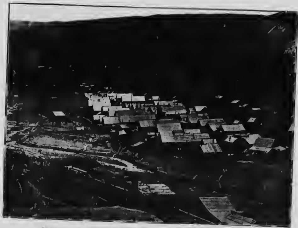
BARKERVILLE, WILLIAMS CREEK, CARIBOO, BEFORE THE FIRE.
