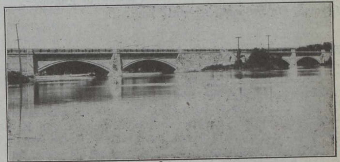
Downstream Elevation, Lemieux Island Bridge
