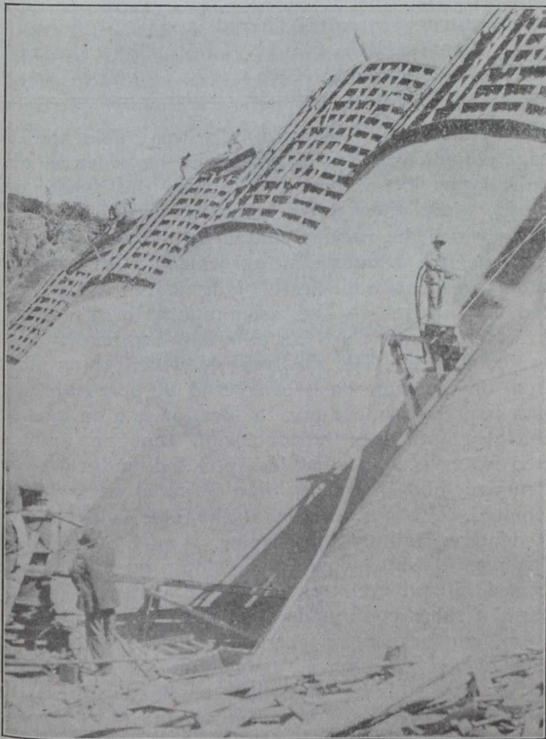
Fig. 3.—Guniting Arches on Gem Lake Dam, Using Cement-Gun
