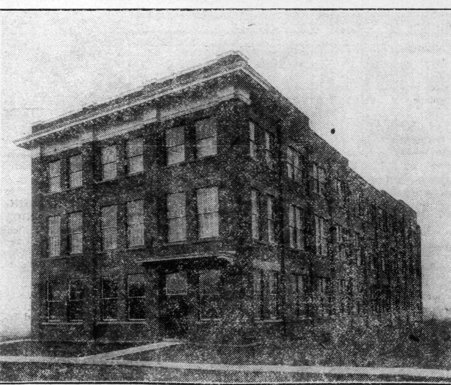
Building of the Niagara Silk Company, Limited
