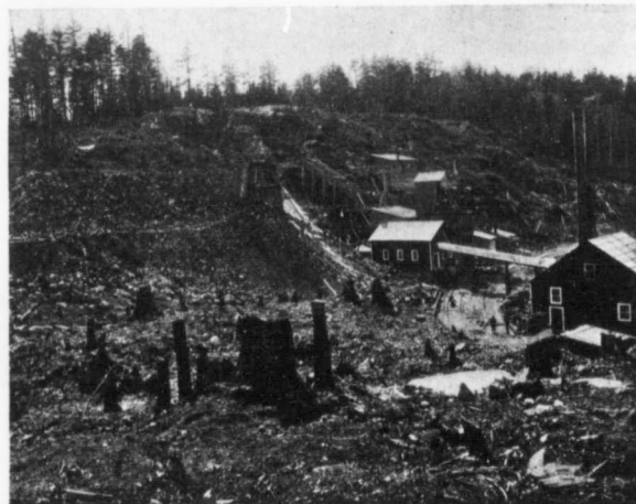
The Power and Crushing Plant, Open Pit and Ore Stock Pile, Moose Mountain Mines.
