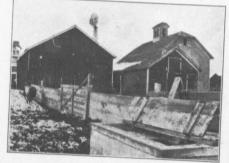
A Concrete Fence for a Windbreak A concrete fence such as the one here illustrated, the construction of which is described in the adjoining article, is of decided advantage on the live stock farm, affording as it does a shelter from wintry winds during the exercising hour.
