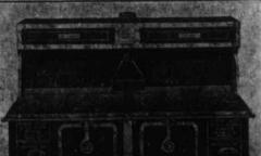
Can be made in sizes to suit the smallest Restaurant, or largest Public or Private Institution. Ovens are deep, wide and high, af-fording large baking capacity. They are fitted with patented Heat controlling dampers
