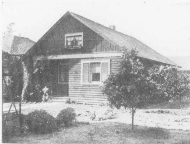
Clapboards differ but slightly in appearance from the overlapped boards, but they are narrower. The cost was \$700
