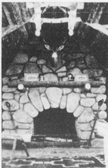
A very good piece of arch work with large stones and raked-out joints. Notice the shelf of a half-log supported on log pins
