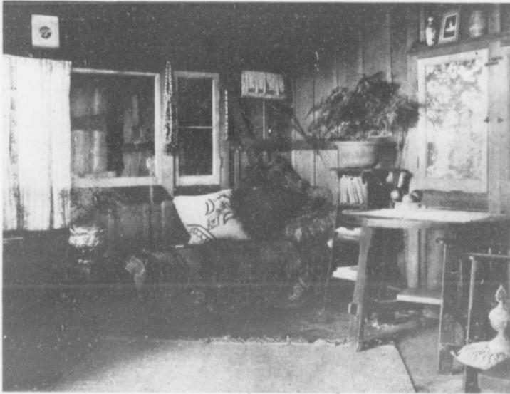
An inside finish of battened boards is used here, giving the effect of being set back so as to leave the studding frame slightly projecting
