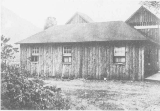
The best way to secure the effect of a log structure inexpensively is to nail slabs—the outside slices of a log—directly to a stud frame
