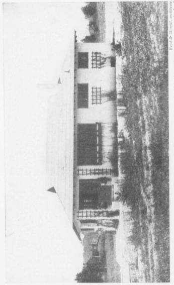
A bungalow at Virginia Highlands, near Washington, D. C., in the building of which the rather uncommon method of pouring the concrete into molds was employed. The cost was \$2,000. Latticework and vines give attractive spots that are well placed
