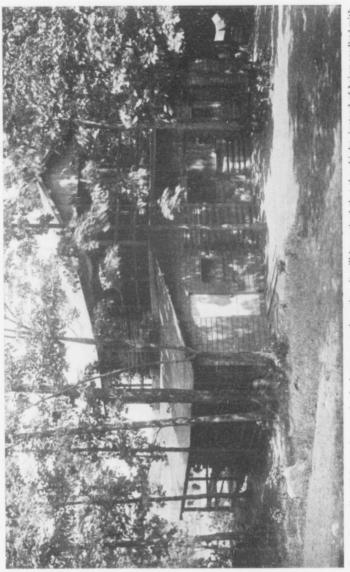
In the log wall, which may be seen in the lower central portion, it will be noticed that the chinks, instead of being caulked with plaster or some material of that sort, are filled with small saplings wedged into place. Most of the upper portion of the shack is used as a sleeping-porch
