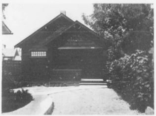
The side walls of shakes are carried directly down to the ground—a rather unusual form of foundation excepting in cheap construction. This whole bungalow cost but \$1200. It consists of five rooms and a bath
