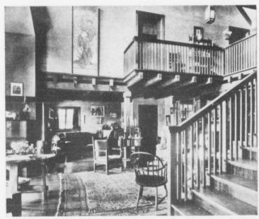
An interesting effect has been secured by leaving the floor joists uncovered to form the ceiling of the first story. The balcony is supported on these floor joists as cantilevers
