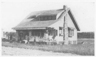
Brick piers are used here, with stone for the chimney. Whatever piers are used, latticework should close the openings between them
