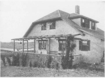
There is an excellent suggestion here in the Haynes house for a method of building porches that will not cut off light from the most important rooms of the house. The framework may be covered by a roll awning when desired
