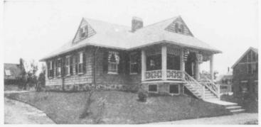
A continuous wall of stone has been used, with a raised line of pointing on the outside. The latter would be out of place with a less finished style of summer home
