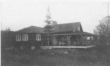
Rough hemlock boards, nailed vertically from sill to plate, with battens on the outside, are used for the walls. The cost of the bungalow complete was \$1500
