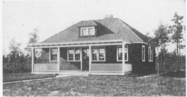
Rough boards laid horizontally over the studs are used in this bungalow at Brightwaters, Bay Shore, L. I. The plan consists of living-room, kitchen, five bedrooms and bath
