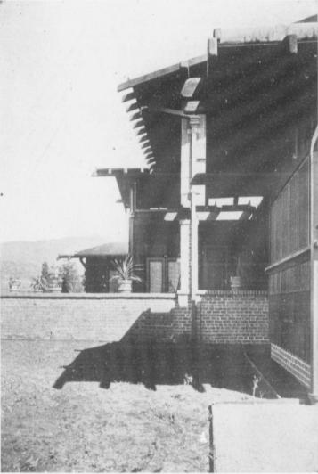
Other exteriors on pages 37, 114; interiors on pages 145, 151 Geo. A. Clark & L. du P. Millar, architects. The roofing is turned over a rounded edge at the eaves in a way that gives it the appearance of a solid lead roof. The roof rafters inside are sheathed, the spaces between them being filled with sawdust to keep out the heat
