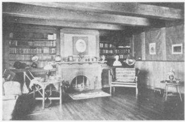
The walls are finished with a perfectly plain wainscoting of cypress, above which burlap is used between the upright strips under the boxed ceiling beams
