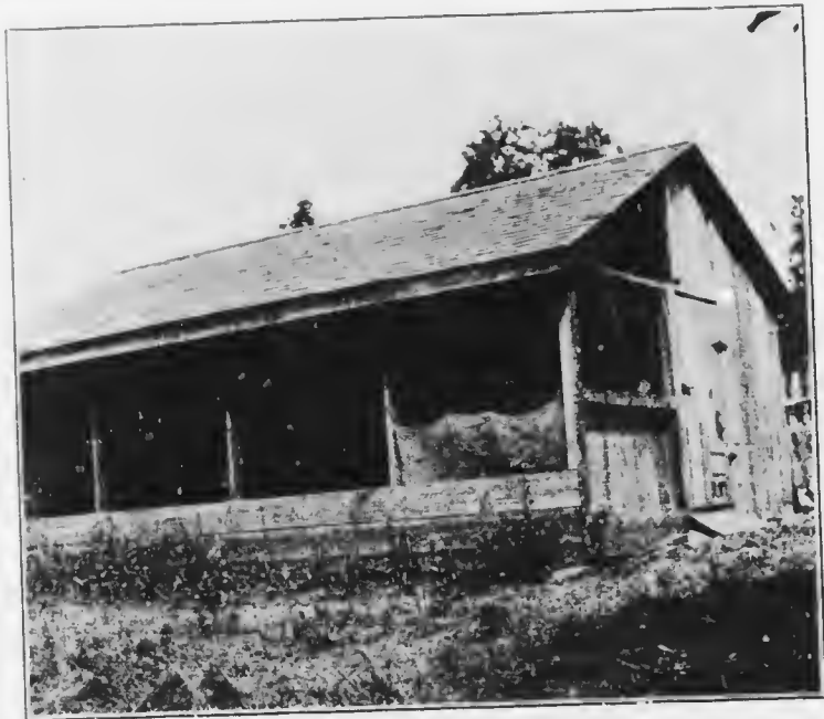
Showing a poorly constructed wall. Openings such as are shown in this cut allow too many draughts.
