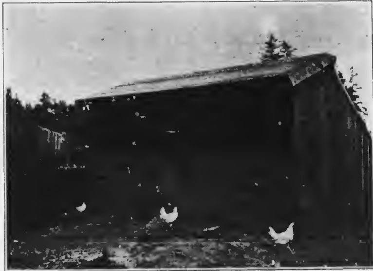
A 12-inch board (1 x 12 inches) at the top of the opening would be of service to keep the temperature more even inside.
