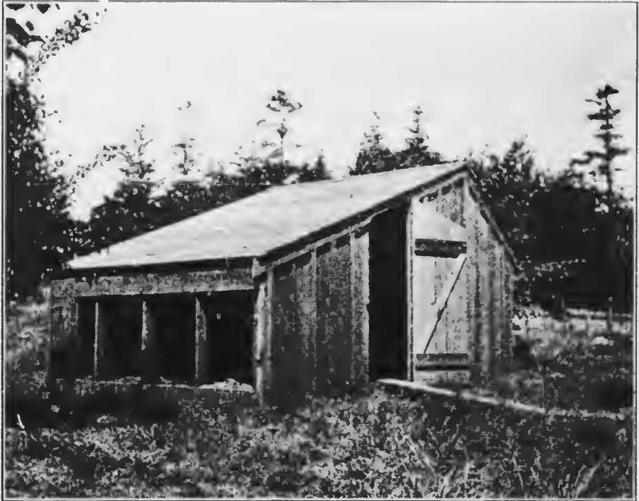
Cut showing Tolman open front arrangement.
