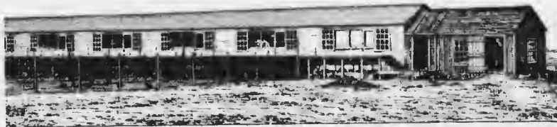
To show the glass arrangement in place of all wood.
